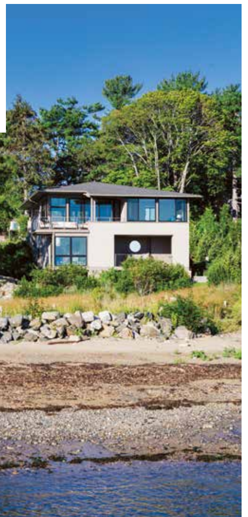
ABOVE: The pool-facing facade's generous overhang offers protection from the hot sun. RIGHT: Ample fenestration on the ocean-facing side affords breathtaking marine vistas and glimpses of the beach. FACING PAGE: A balcony off the living room cantilevers over the rock ledge facing the ocean.
